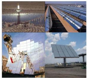
Figure I-1. CSP Technologies (from upper left, tower, trough, dish-Stirling, and CPV)
