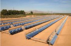
Fig. I-6. Final stages of installation of trough solar field at the 1MW APS
